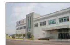
Tractor Engine Plant
